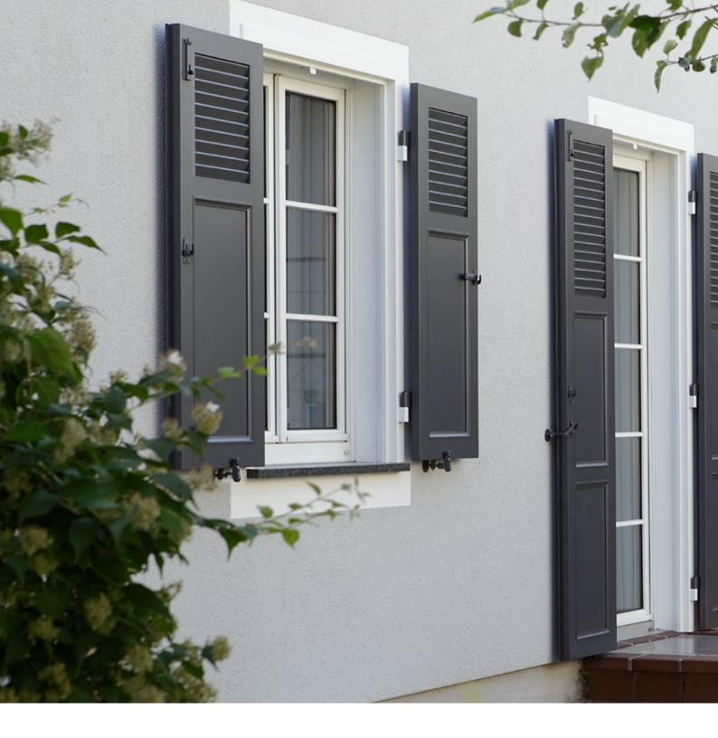
EHRET installation frames connect shutters to the façade. In the area of the wall opening, the frame supports the wall reveal on at least three sides. In doing so, aluminium frames not only have important technical functions but also make for a design highlight on the façade as they come in a variety of colours.
