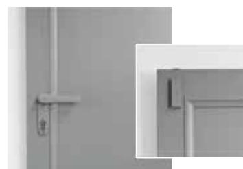
Rod lock (installed)
